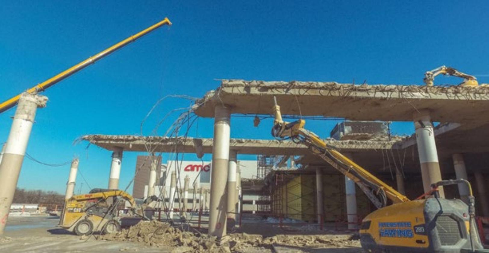
Two robots were operating at the same time during each 10-hour shift. The area was surrounded on three sides by an operating shopping mall.
