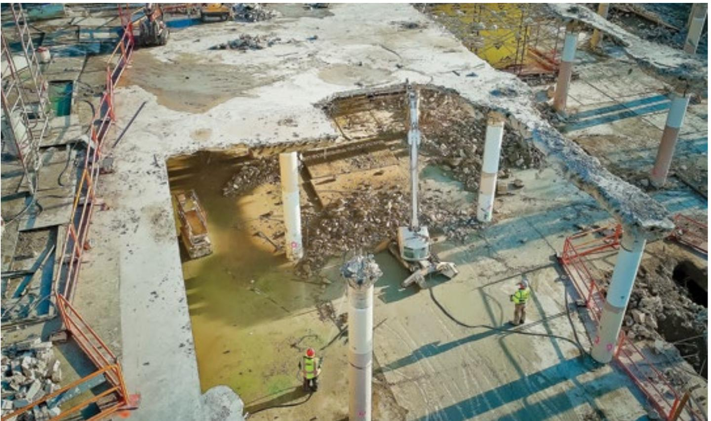
Two floors of an old Sears department store were demolished by crushing and removing the concrete.
